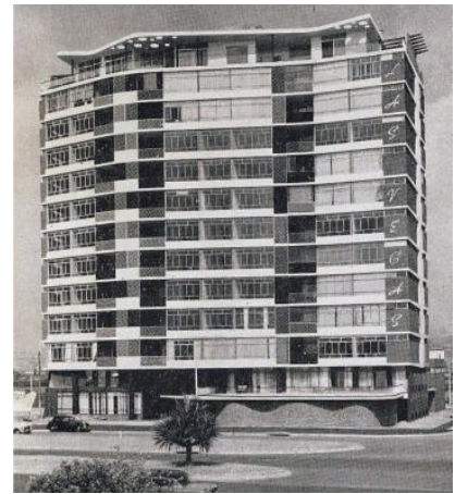
Fig. 5.3.3- Photograph of Las Vegas apartment block taken from the boulevard (Source- Benjamin & Crofton: 1958, 36)
