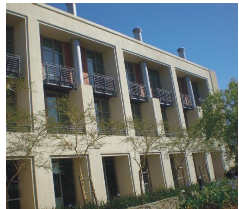
Fig. 5.5.3- Photograph of the SE elevation depicting the recessed windows created by the ventilation stacks (Source- By Author)
