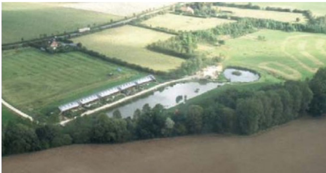
Fig. 4.2.5- areal photograph of Hockerton Housing Project (Source- Energy Saving Trust: 2003)
