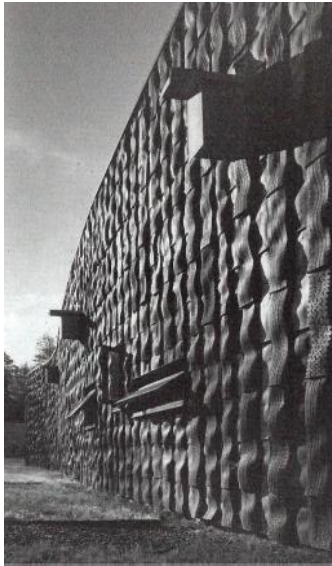
Fig. 4.2.14- Detailed photograph of the tireclad wall at the entrance of Pocono Education Centre (Source- Moskow: 2008, 61)
