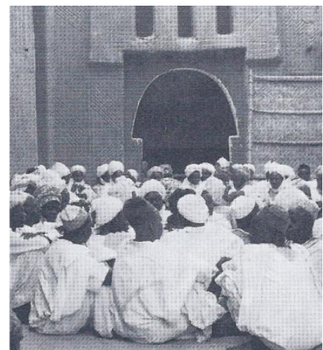
Fig. 3.2.14- Photograph of a courtyard at Hausa Palace, Nigeria used for social gatherings (Source- Denyer: 1978, 177)
