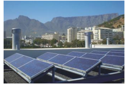
Fig. 5.5.9- Photograph taken from the roof of the PV panels (Source- By Author)
