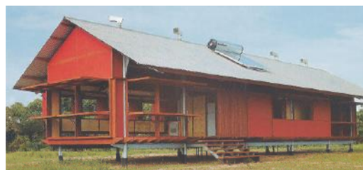
Fig. 4.3.26- Photograph of Marika-Alderton House illustrating cross ventilation techniques and rotary turbine vents (Source- Fromonot: 2003, 219)
