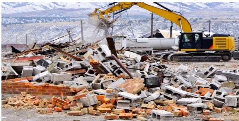
Figure 2.1: C&D waste in a construction site (Source: (Pinatih, 2020))
