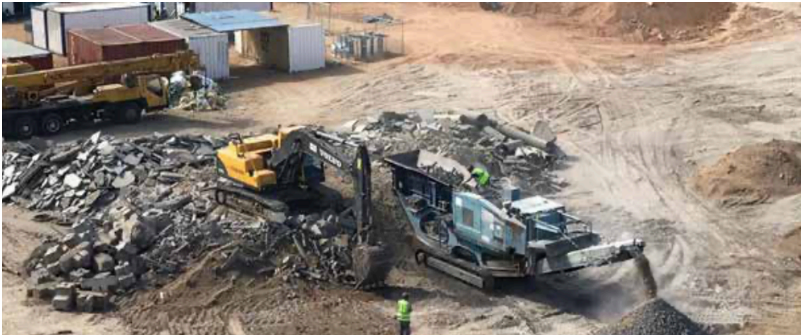
Figure 2.14: Woolworths Distribution Centre site in Montague Garden, Cape Town(Source: GreenCape, 2018b)
