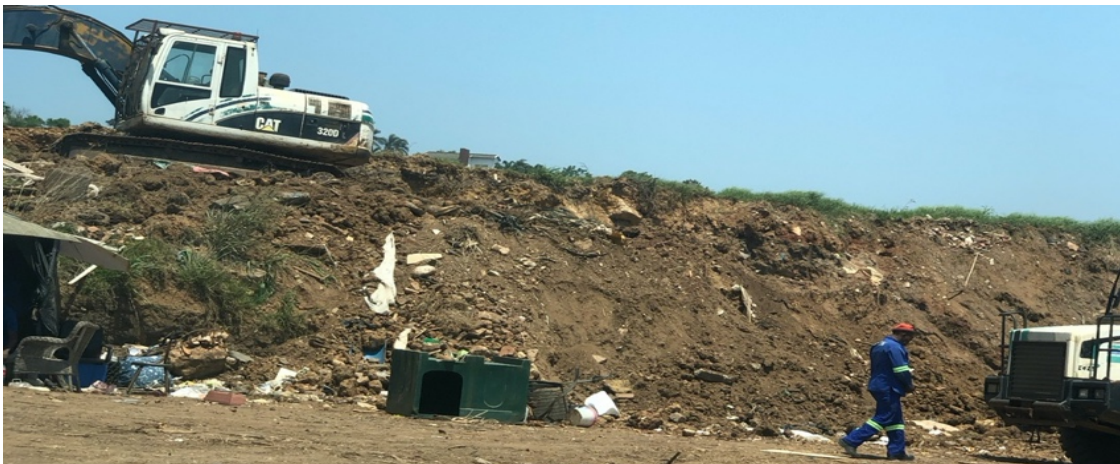
Figure 4.11: Working face at DSW landfill
