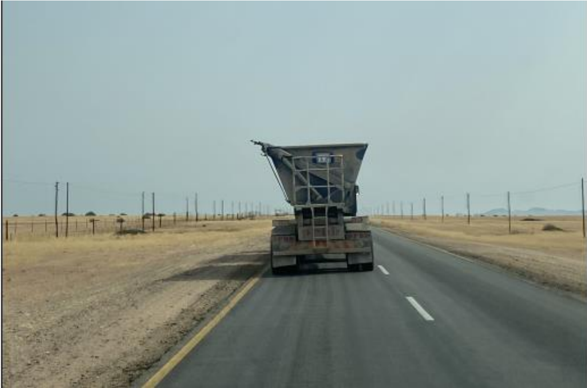
Figure 5-3: Narrow Road widths due to the lack of road shoulders
