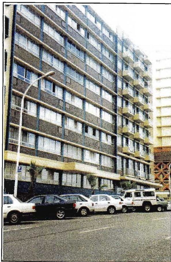
Photograph 2 : Hawaii Apartments West Block
