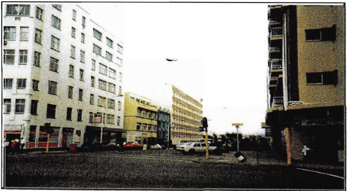
Photograph 5: Surrounding Buildings (Point Road)
