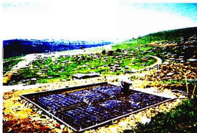
Figure 6 : Damp proofing and steel reinforcement of foundation.
