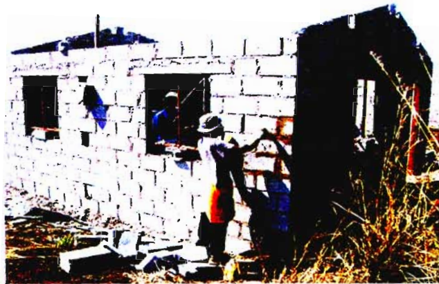
Figure 11 : Joints being filled and internal wall construction.
