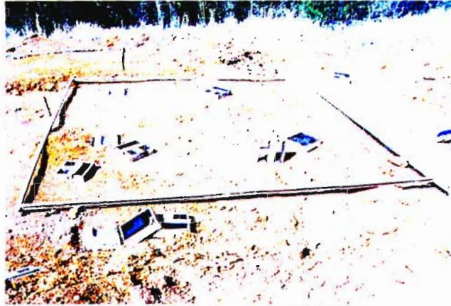
Figure 4 : Preparation for constructing foundation.
