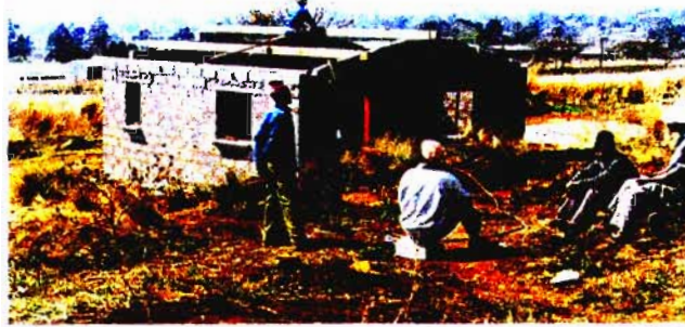
Figure 13 : Roofing of structure commencing.
