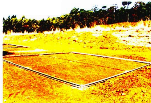
Figure 5 : Preparation for foundation continued.
