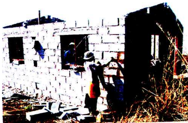
Figure 11 : Joints being filled and internal wall construction.
