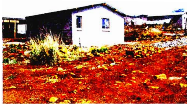
Figure 14 : Completed unit ready for occupation.
