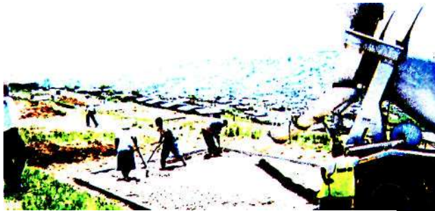
Figure 7 : Pouring cement for foundation and slab.
