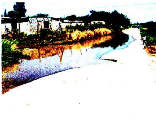
Figure 17 : Poor service maintenance.
