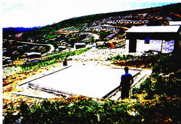
Figure 8 : Slab completed, ant poison applied and clearance commencing.
