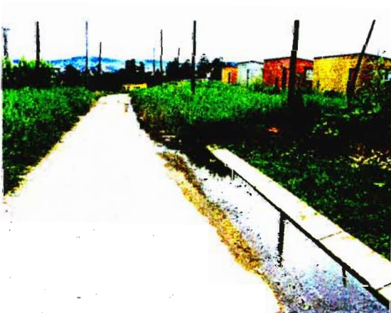
Figure 15 : Poor service maintenance.
