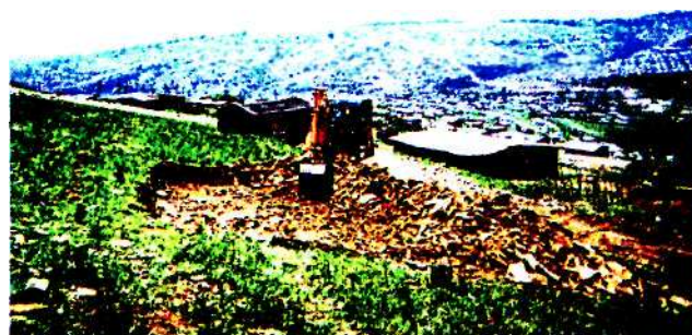
Figure 2 : Platform excavation for foundation.
