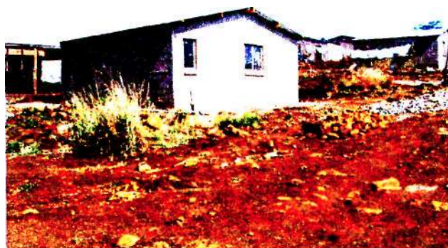
Figure 14 : Completed unit ready for occupation.
