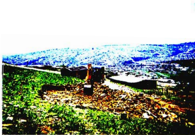
Figure 2 : Platform excavation for foundation.
