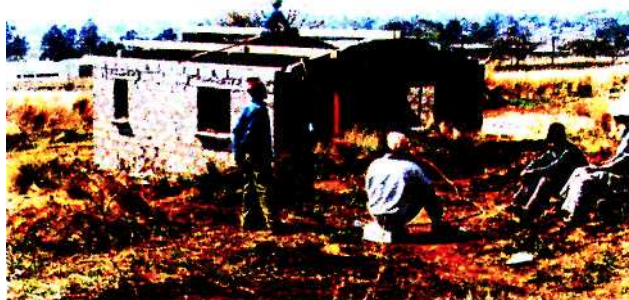
Figure 13 : Roofing of structure commencing.
