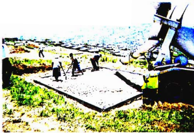
Figure 7 : Pouring cement for foundation and slab.
