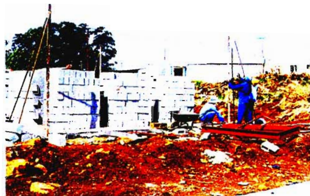
Figure 9 : Setting profiles to construct walls.
