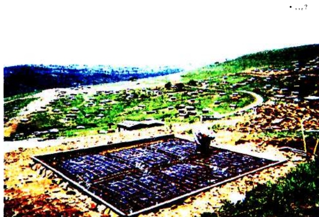
Figure 6 : Damp proofing and steel reinforcement of foundation.
