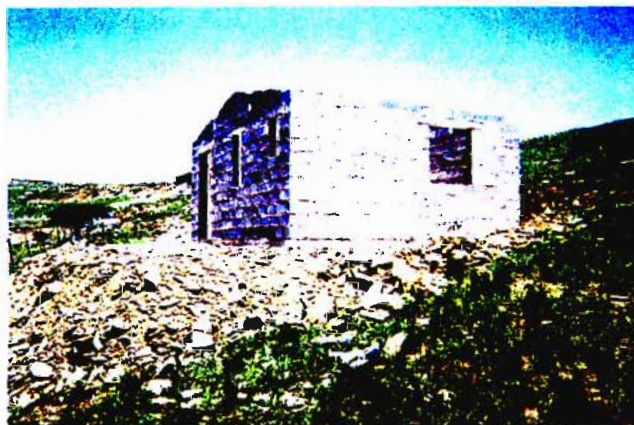
Figure 12 : Unit completed to plate level.
