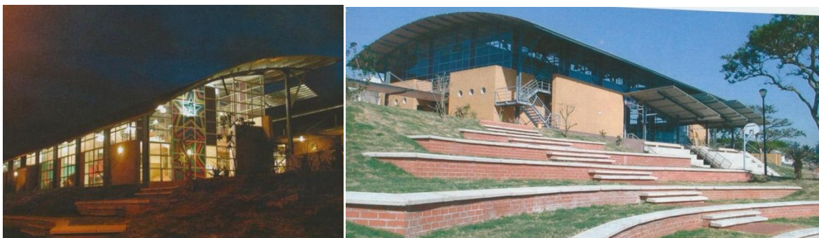
Figure 45 External views of youth Centre (Digest of South African Architecture, 2004/2005: 78 &79)
