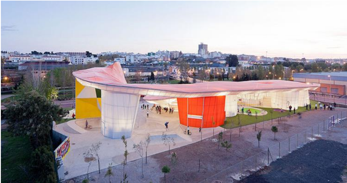
Figure 36 The orange roof sweeps over the entire centre as a symbol of unity and protectiveness. (www.fastcodesign.com)
