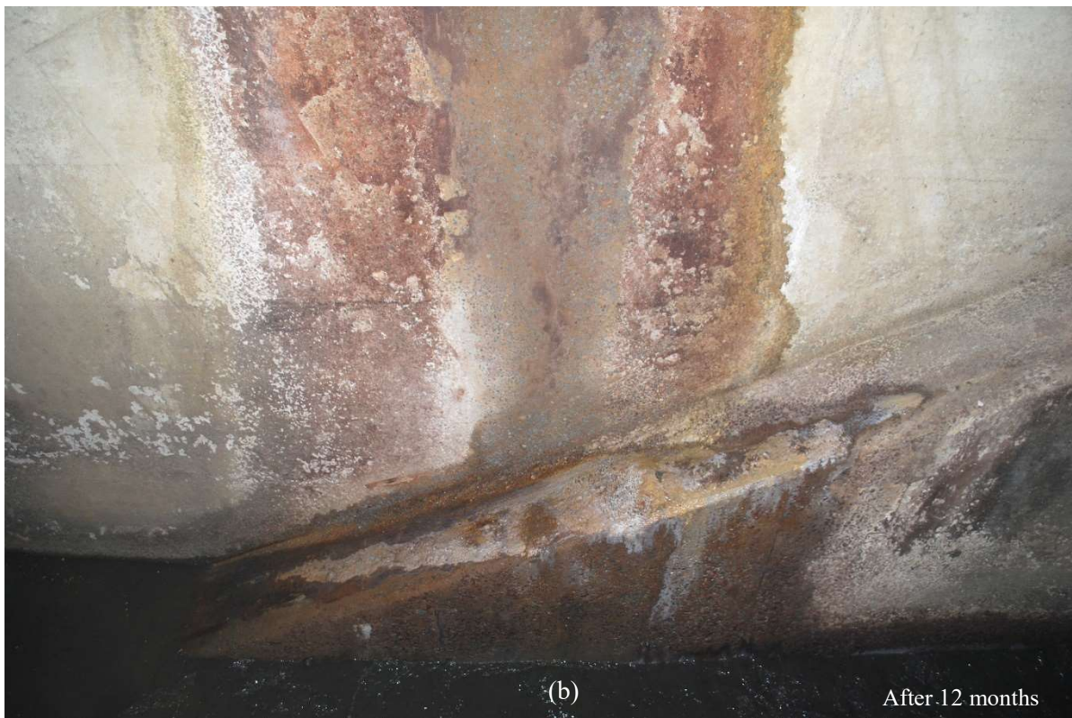
Figure 4-5: Progressive effect of MICC at the exposure site
