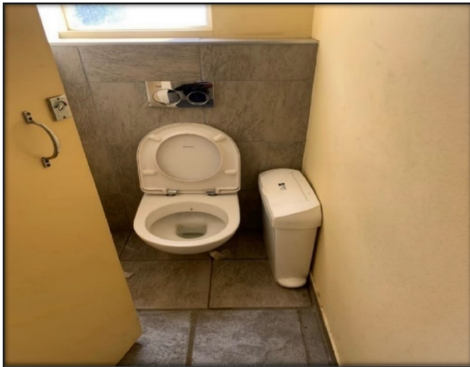
Figure 6.42. College C: Ablution Facilities—Female Toilet Stall
