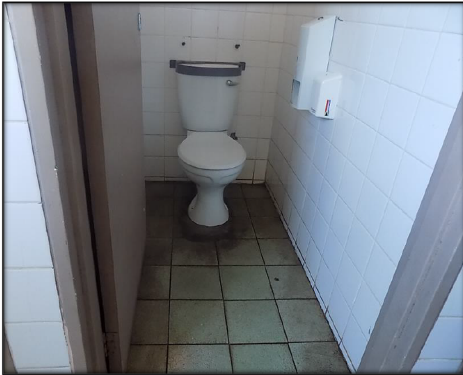
Figure 6.29. College B: Ablution Facilities—Toilet Stall
