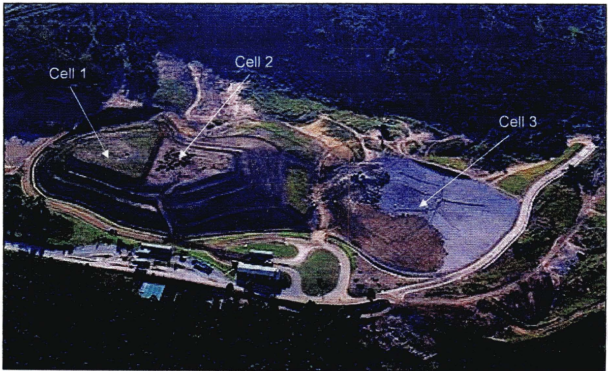
Plate 5.3 Aerial view of the Mariannahill Landfill Site, showing the location of the three cells (Courtesy DSW)
