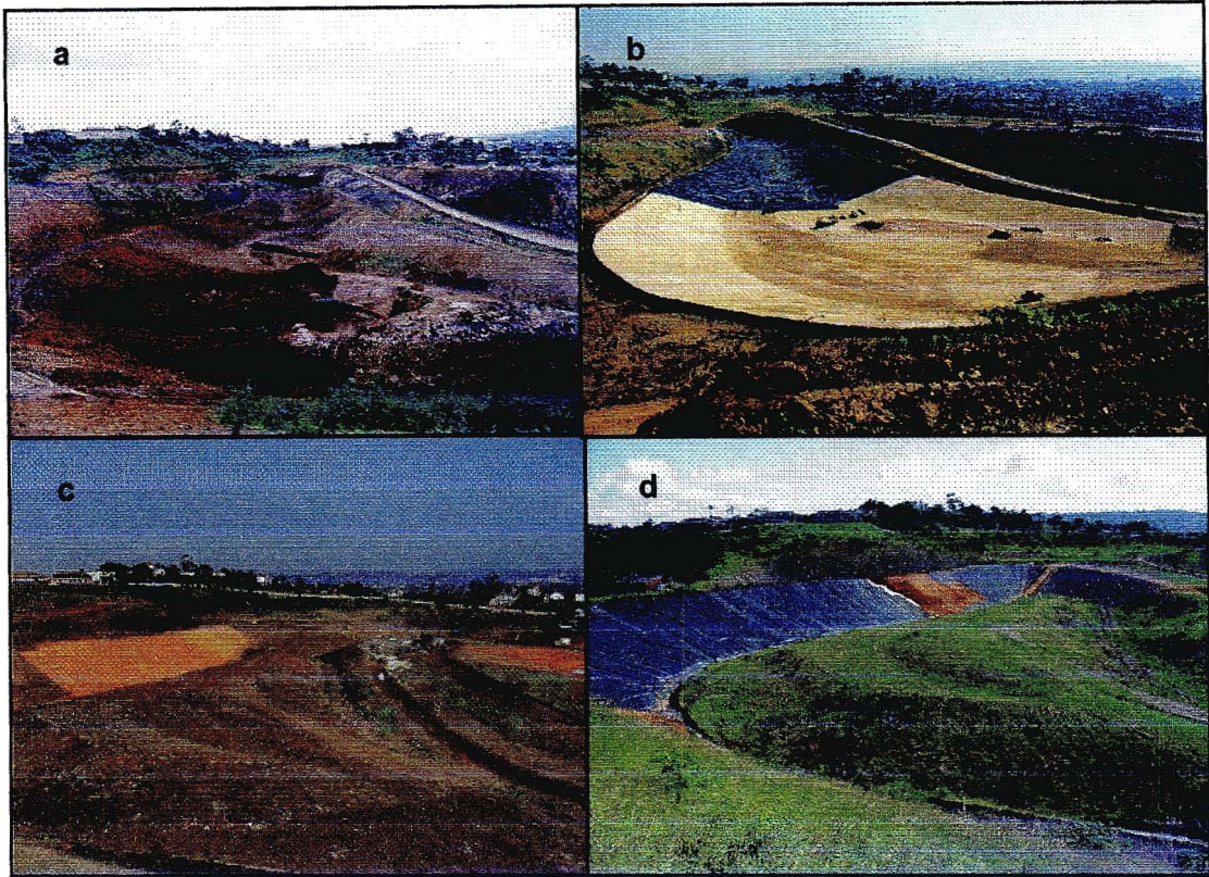
Plate 2.1 The progression of a landfill cell illustrating the method of Cellular Landfilling – a) Preparation of cell; b) Lining of cell; c) Filling of cell; d) Closure of cell.
