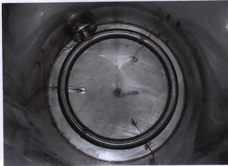
Figure 3.15 Steam manifold.
