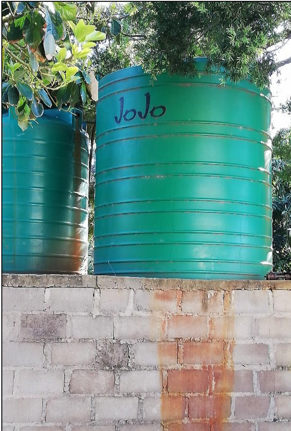
Figure 0.6. Water preservation for the community in Ward 11, uMhlabuyalingana LM
