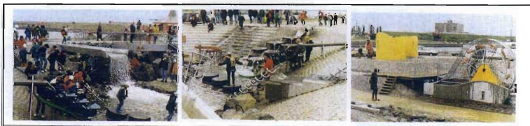
Figure 13: showing construction of the water park (Zevi: 1996, p.455)
