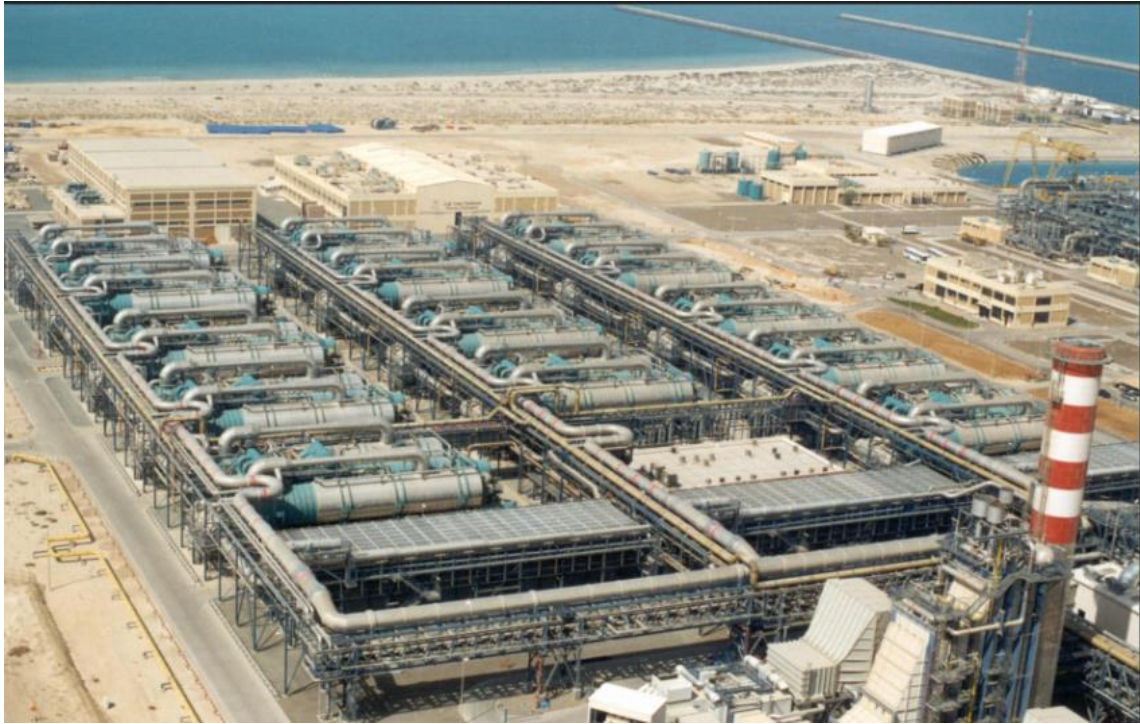
Figure 2.1: Desalination plant in Saudi Arabia (Utilities middle east, 2018)
