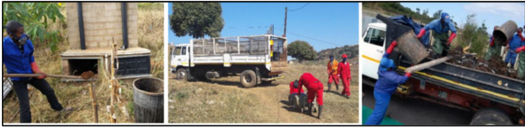
Figure 2.3: The emptying and transportation of faecal sludge from UDDTs.
