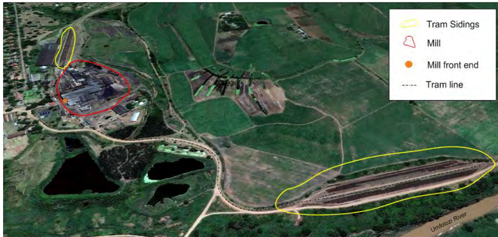
Figure 3.3 Umfolozi Sugar Mill and tram sidings where the stockpile will be created.
