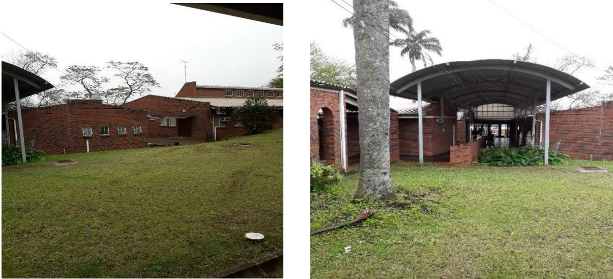
Figure 1.1 The southern, eastern and western view of the centre.
