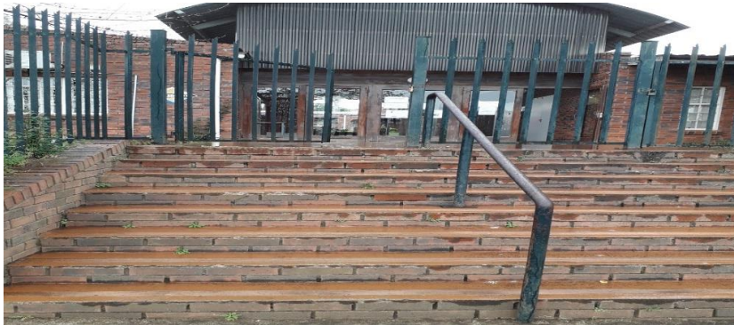
Figure 1.6 The main entrance showing palisade fencing and razor wire.
