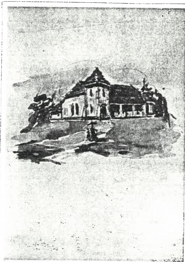
w48 [BUILDING] - 1916, p. 265
