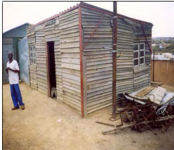
Figure 9: Framed house in Illovo after it has been extended with poor quality building materials
