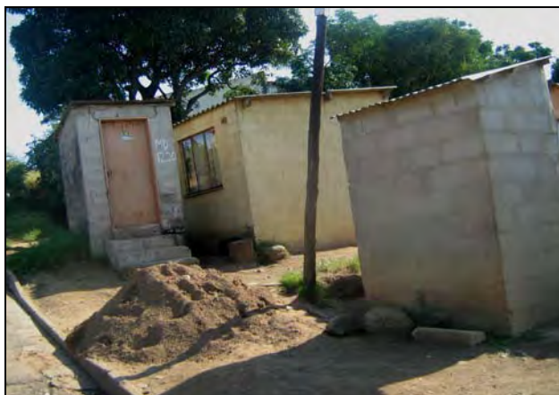
Figure 3: Pit latrines in Bester's Camp
