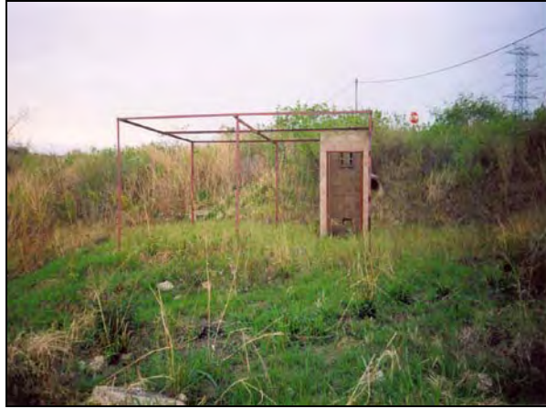
Figure 8: Framed house with a toilet in Illovo Phase 4
