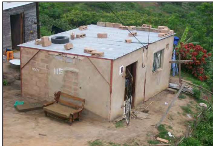
Figure 10: Framed house after it has been built using bricks and cement
