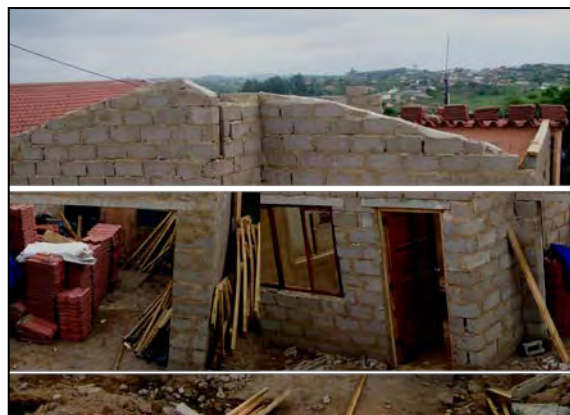
Figure 6: House Extension to Create Enough Space in Illovo.
