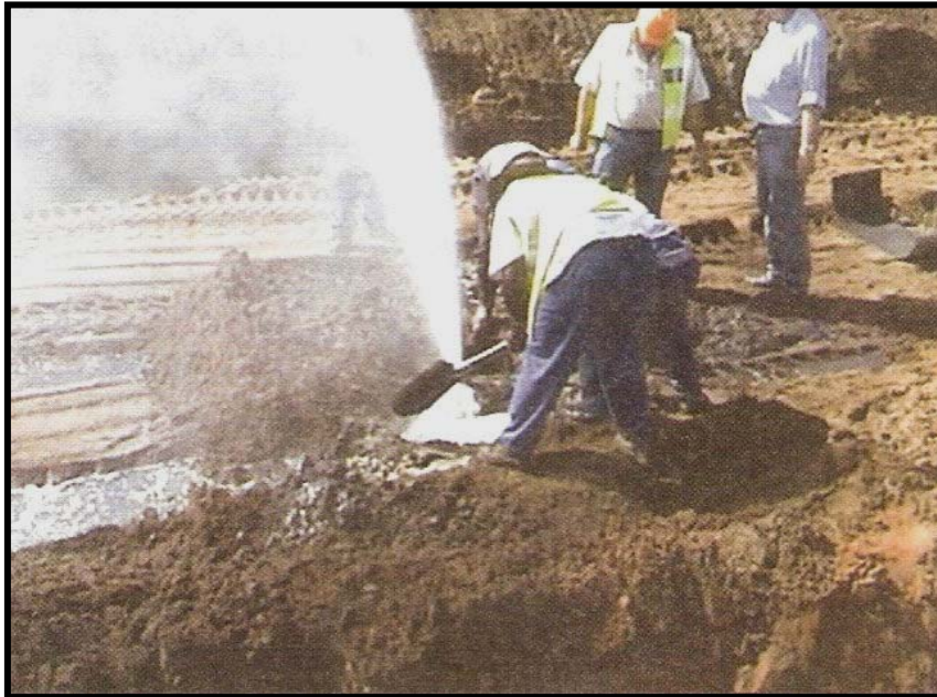
Photograph 12: Burst Pipeline during a SAPREF pipeline replacement project
