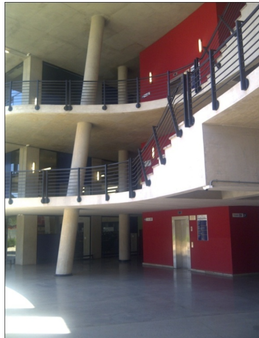
Plate 6.5 The irregular columns within the Wits science stadium (Authors own image)
