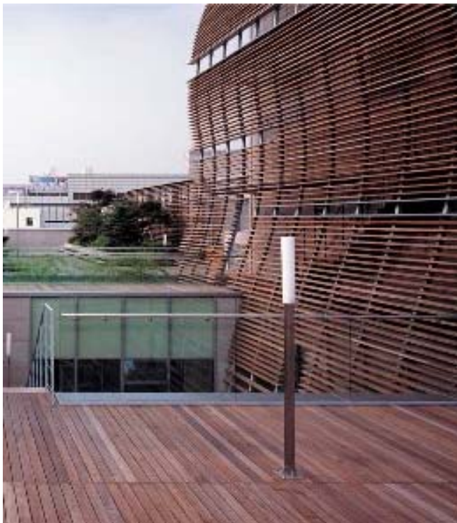
Plate 3.12 The curvilinear aesthetic treatment of the CHA Women and Children's hospital ( www.architectureweek.com/2008/0917 )
