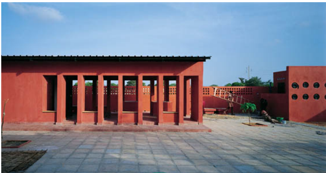
Plate 4.20 The building utilises local building methods and is painted a vibrant red conveying notions of strength. ( www.archithoughts.wordpress.com/2011/03/31/womens-centre-in-rufisque )
