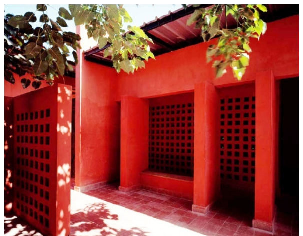
Plate 4.23 The sun screens produce a pattern which breaks away from monotonous and anonymous facades (Varandah, 2004:17)
