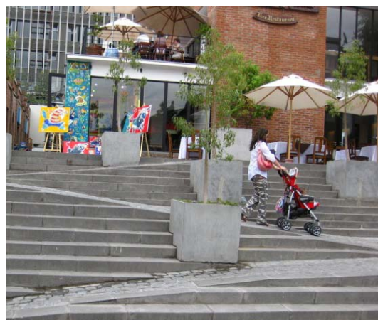
Plate 3.4 A Ramp integral to staircase. ( www.flickr.com/photos/borkazoid/4202740785 )
