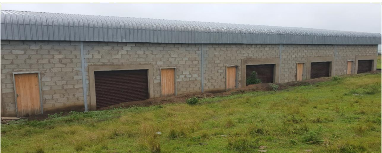
Figure 4.2: Somopho Industrial Park Project
