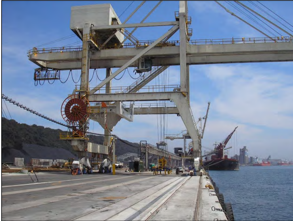
Figure 8: Bulk Connections container crane
