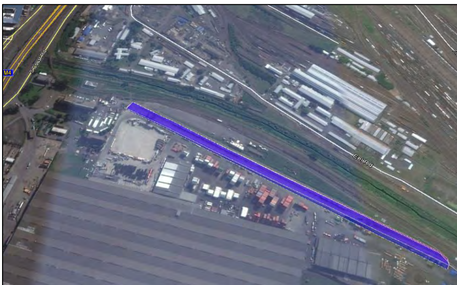
Figure 16: Bayhead rail siding
