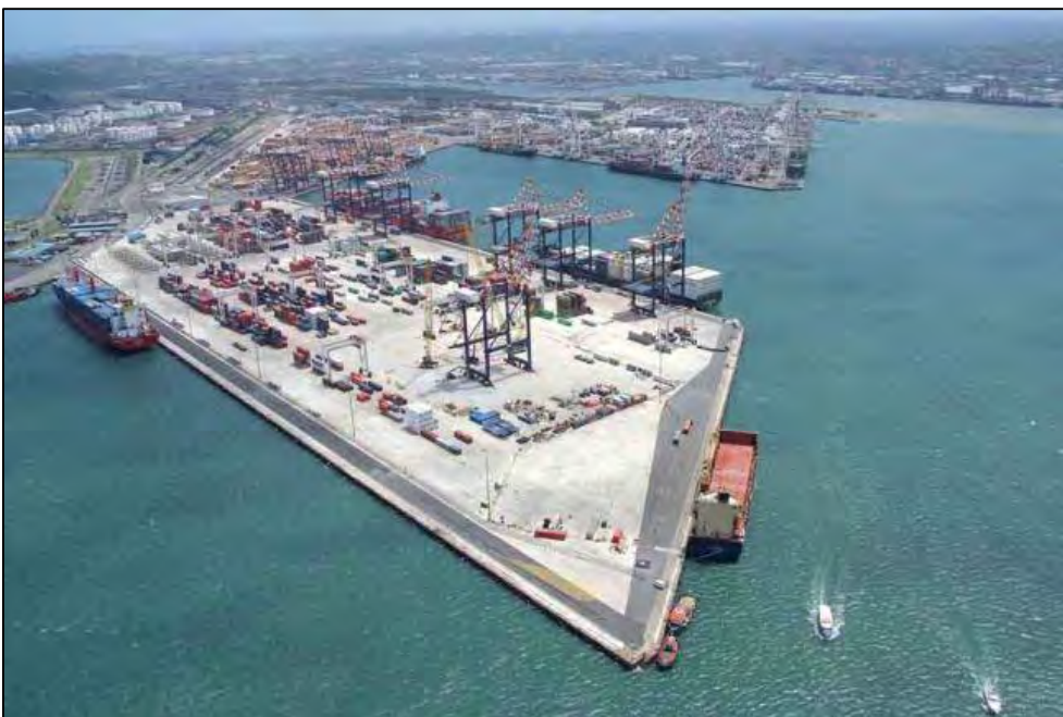
Figure 6: Pier 1 Container terminal
