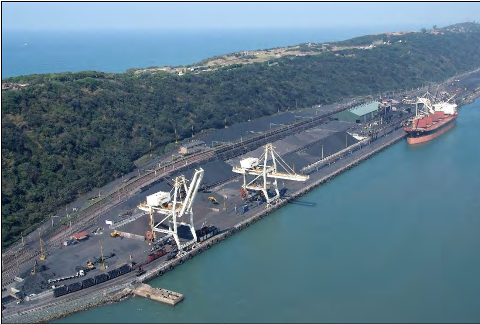
Figure 5: Aerial view of Bulk Connections
