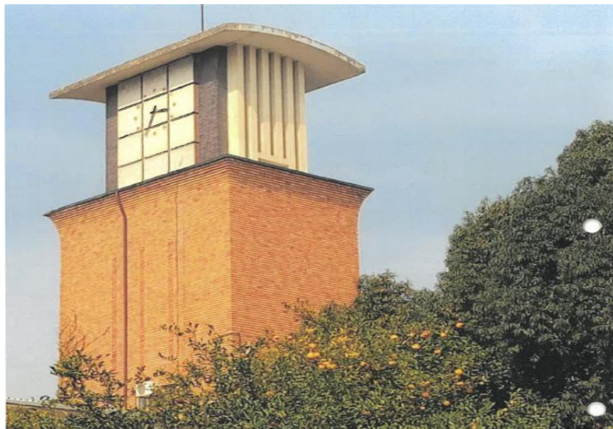
Figure 17: Photograph showing a high tower clock as a symbol of colonial power
