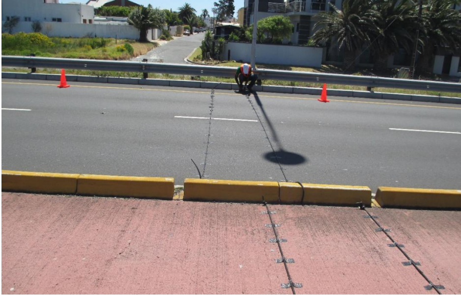
Installation of ATCs and Pneumatic Tubes at SS004
