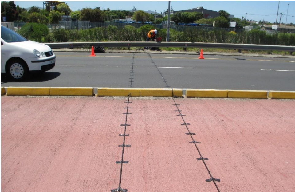
Installed Pneumatic Tubes and ATCs at SS003
