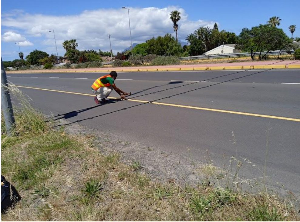
Installation of ATCs and Pneumatic Tubes at SS001
