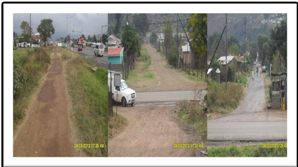
Figure 5.13 Nature of feeder roads in the Edendale corridor section
