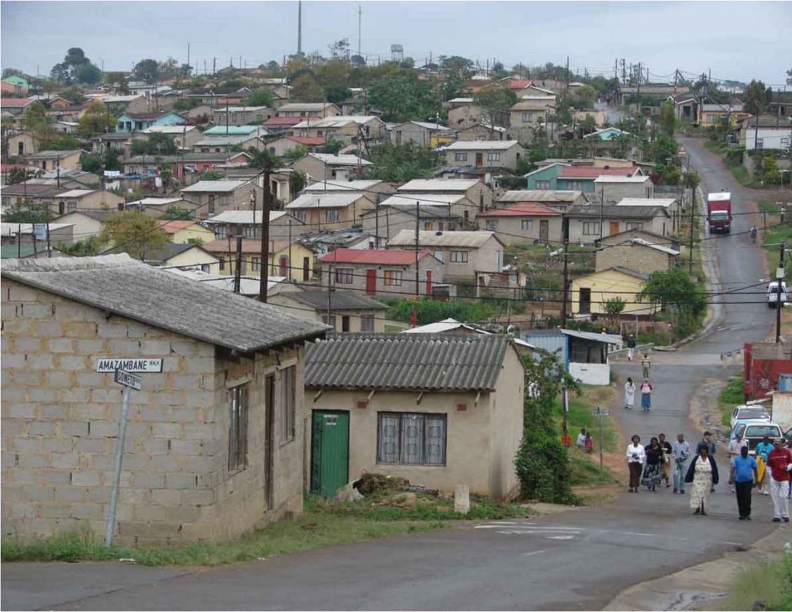
Figure 3: Completed houses of Piesang River Source: Jeff Thomas, (UTshani Fund) 2012
