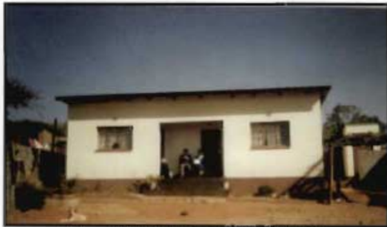
(b) Two rooms with veranda toilet/shower room
