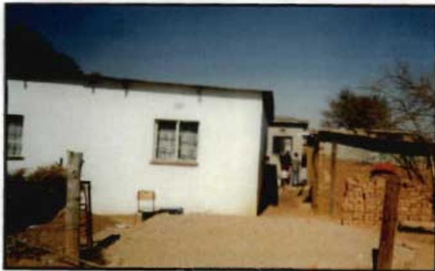
Figure 4.4 Main house, back yard house and 'temporary' mud house
