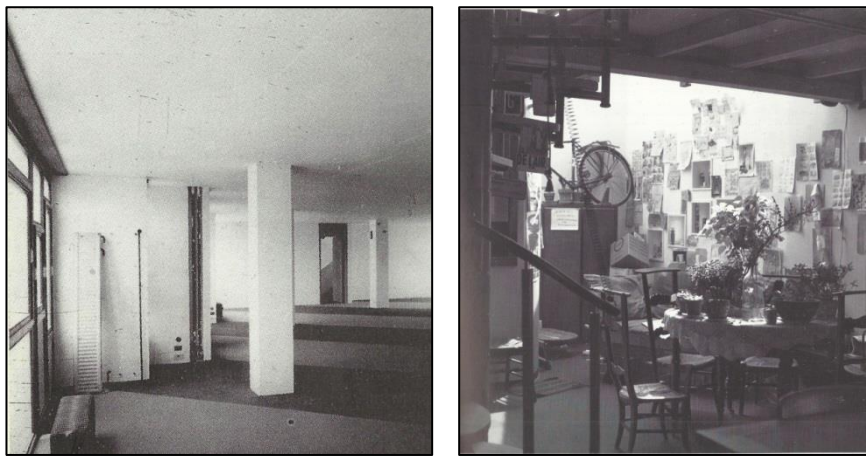
Illustration 5.2.4 (Left) Typical unit floor layout before installation of partitions. (Right) Typical unit after interventions. Source: (Kroll, 1986:48)
