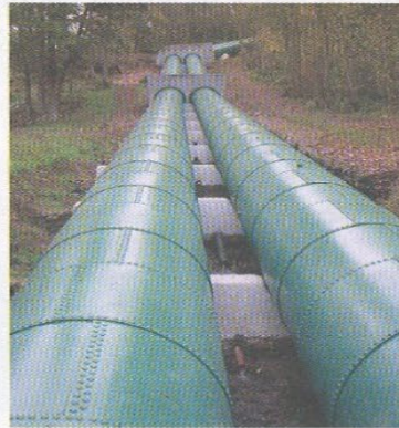
Fig.13.2: Nkula Hydroelectric Station
