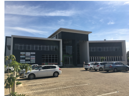
Fig. 3.7. South-east facing main entrance (Source: Author, 2017)
