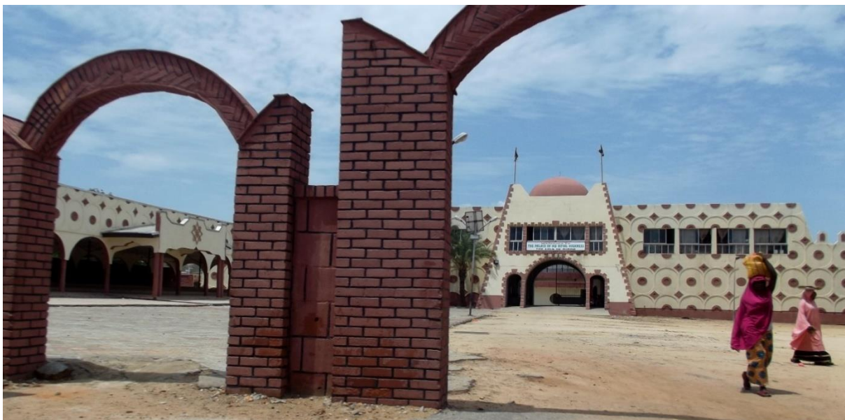
Figure 7.69: Emir's Palace in Minna
