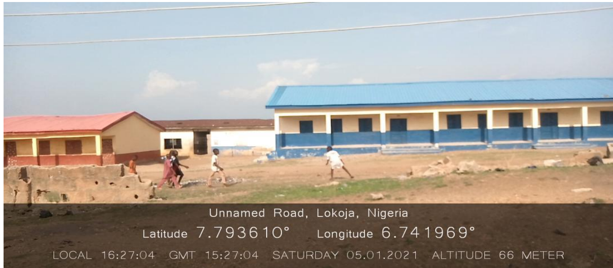
Figure 7.1: Government Secondary School in Lokoja, North-Central Nigeria
