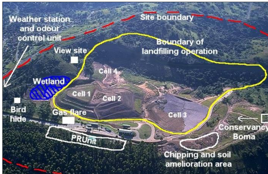
Figure 3: Aerial view of Mariannahill Landfill
