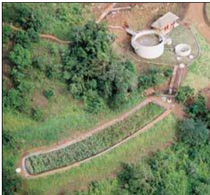
Figure 6: Aerial view of Mariannahill Landfill Site’s Sequential Batch Reactor
