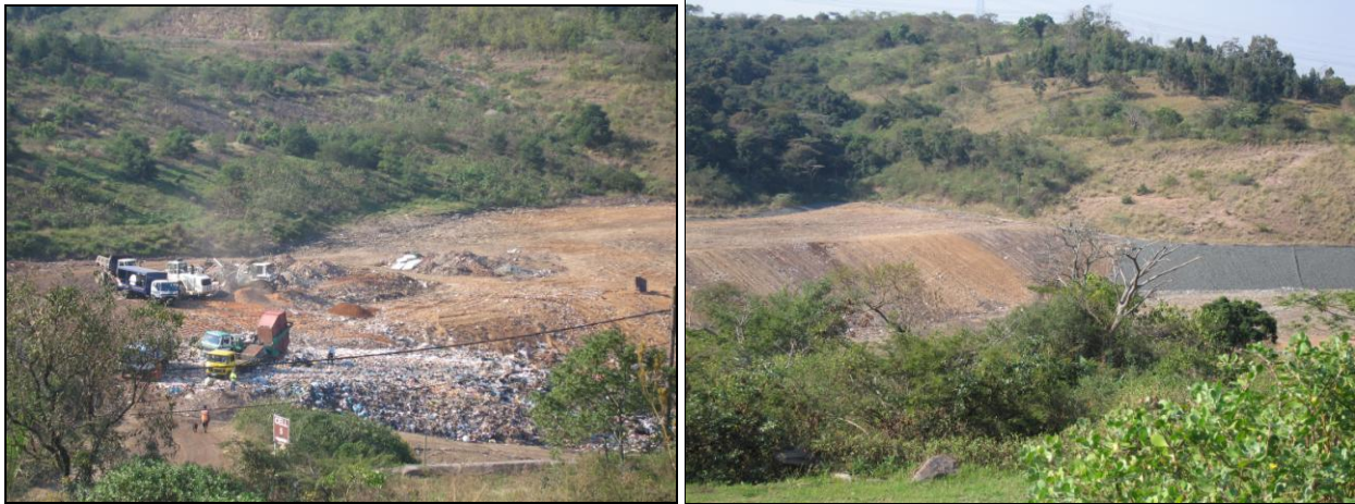
Figure 12: Landfilling, cell re-enforcements and bank stabilization in progress
