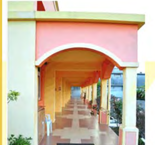
Verandah: functional for shading whilst allowing daylight and natural cross ventilation across the building
