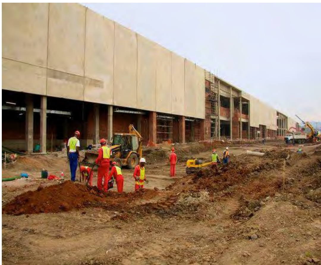
Figure 7: Local People Involved in Construction of Bridge City Shopping Centre (Source: Bridge City Progress-Tracker, 2011)
