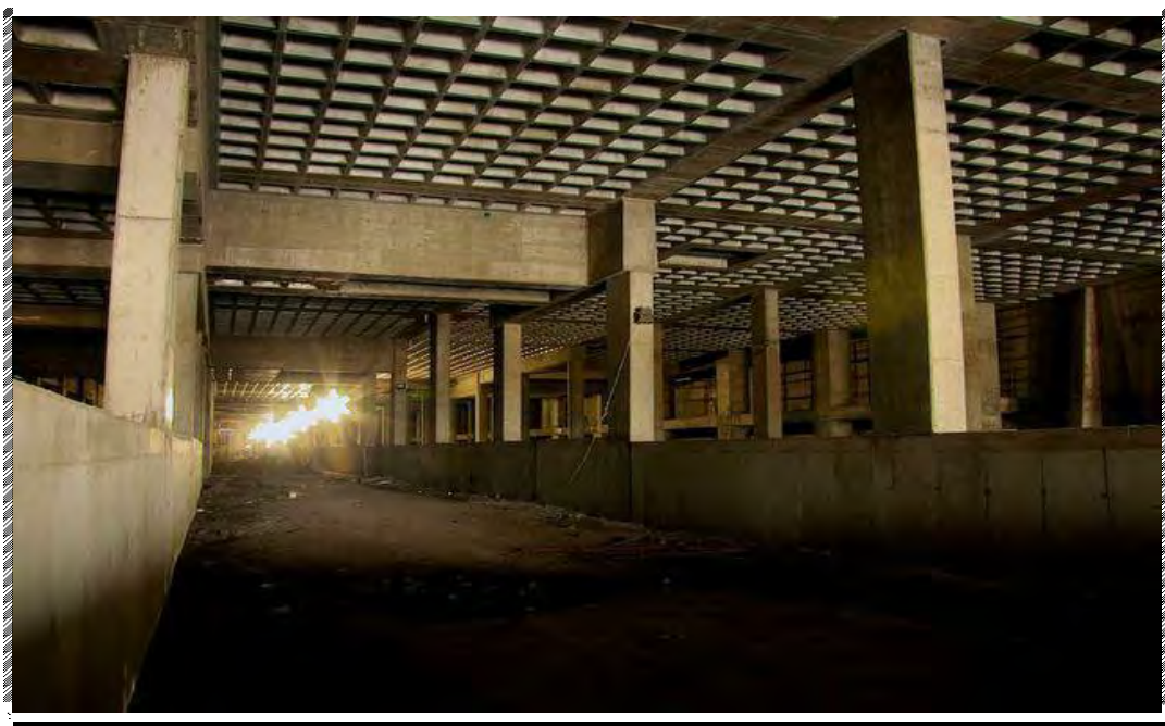
Figure 9: The Bridge City New Railway Station under Construction. (Bridge City, Progress-Tracker (2011))
