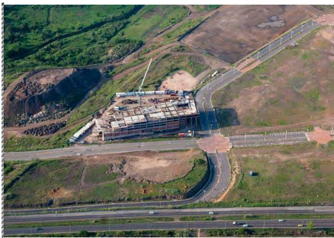
Figure 8: Construction of the Bridge City Magistrates' and Regional Court (Source: Bridge City, Progress-Tracker, 2011)
