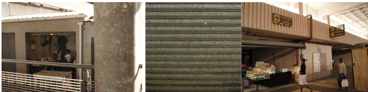
Figure 51: Roller shutter garage doors.
