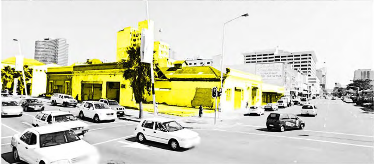
Figure 24: Various views of the existing site conditions and buildings.
