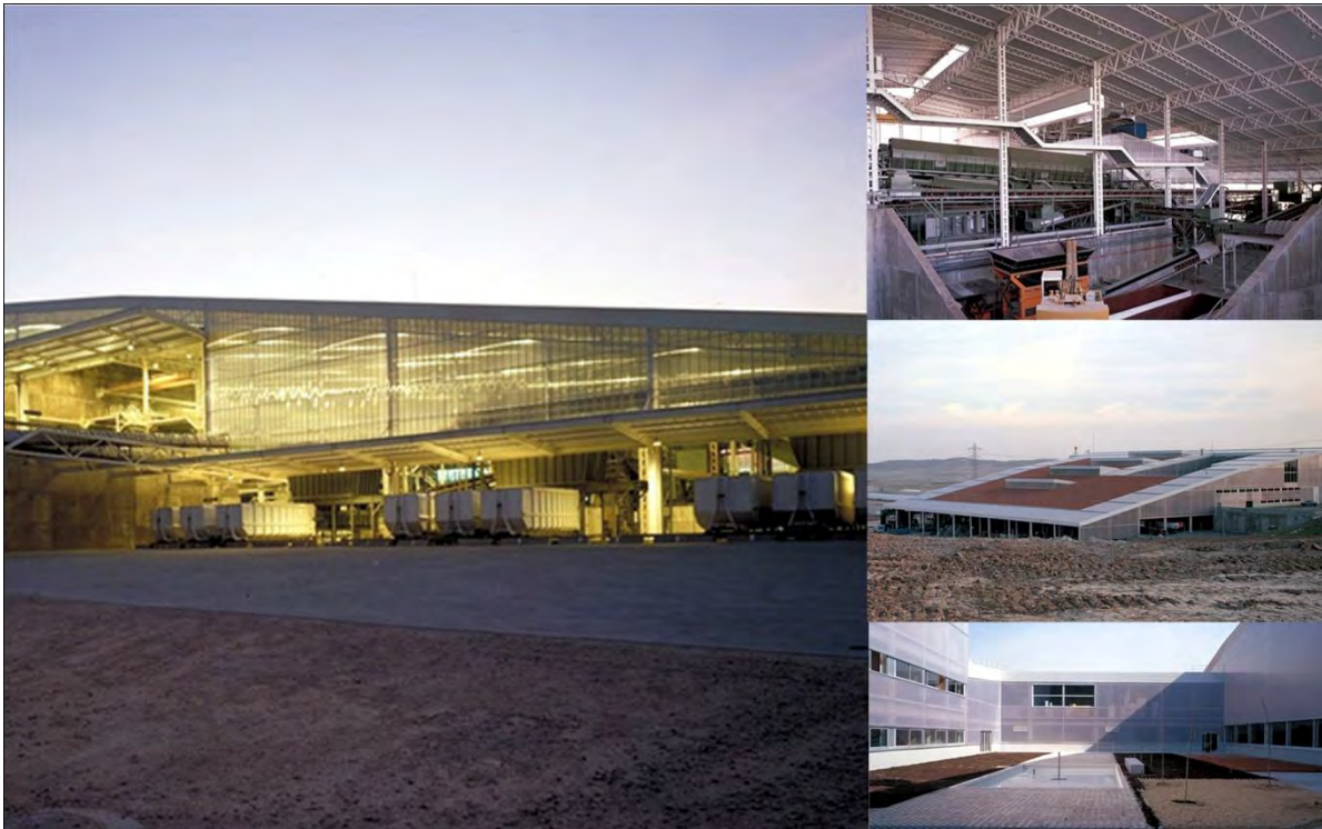
Figure 10: The vast recycling facility at Valdemingomez which was designed to be dismantled.
