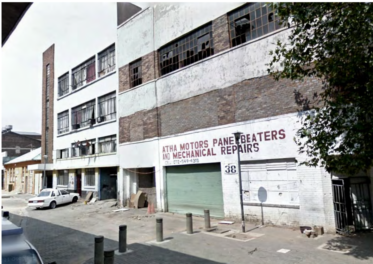
Figure 85-The unassuming, dilapidated House 38 does not suggest the activity that happens within. The mechanic workshop is operational despite the condition of the building and the illegal occupation by the recyclers.
