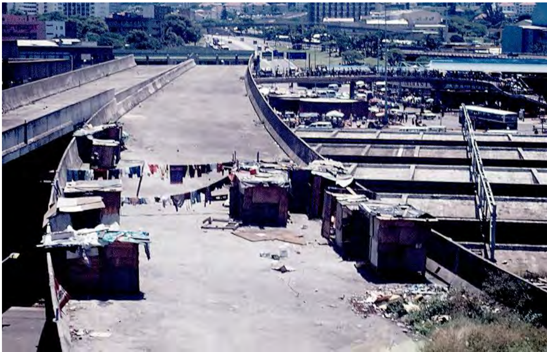
Figure 50-Before the intervention, squatter settlements were starting to be established on the unused freeway spurs, posing health and security risks.
