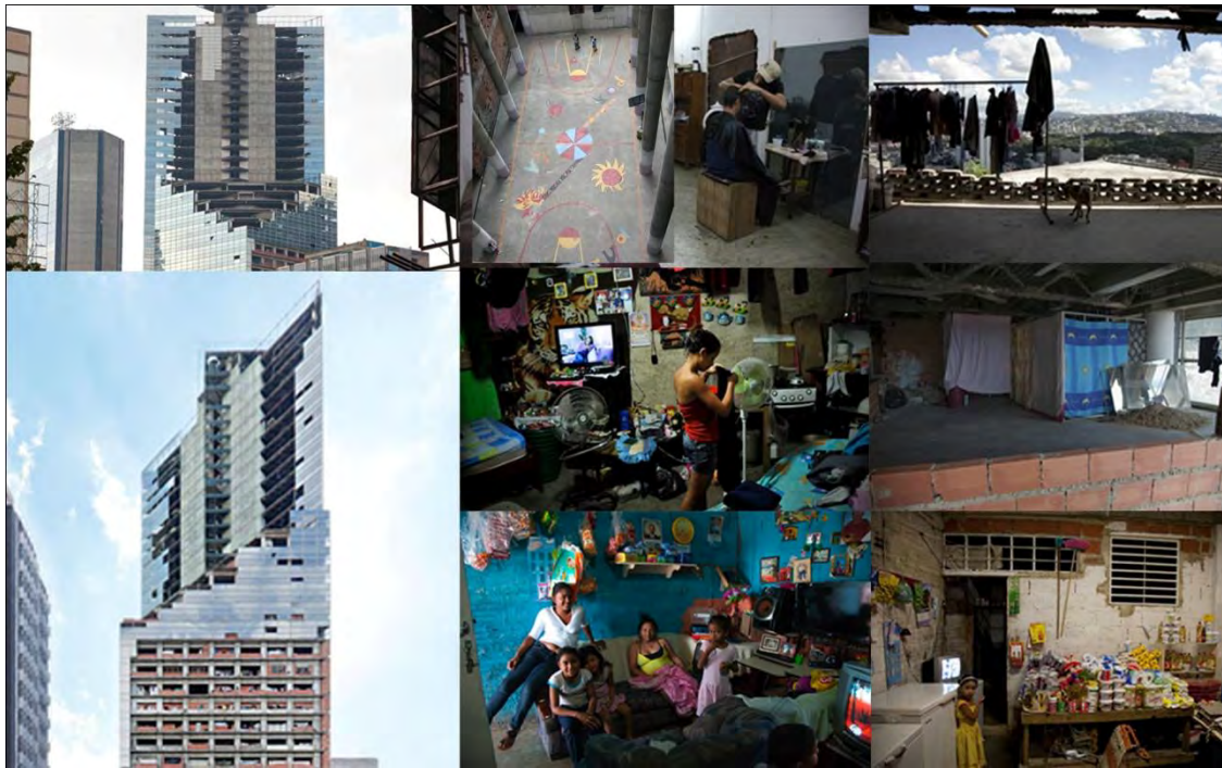
Figure 3: Various views within the so-called Tower of David showing how the insurgent citizens have modified the carcass to create habitable spaces that many call home.
