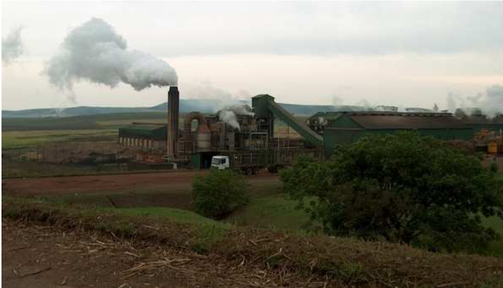
Figure 5.2 A photograph of the Eston sugar mill (Source: Panoramio, 2012)
