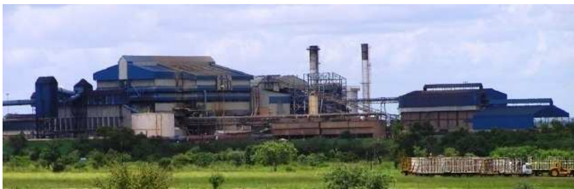
Figure 5.4 A photograph of the Komati sugar mill (Source: Panoramio, 2012)
