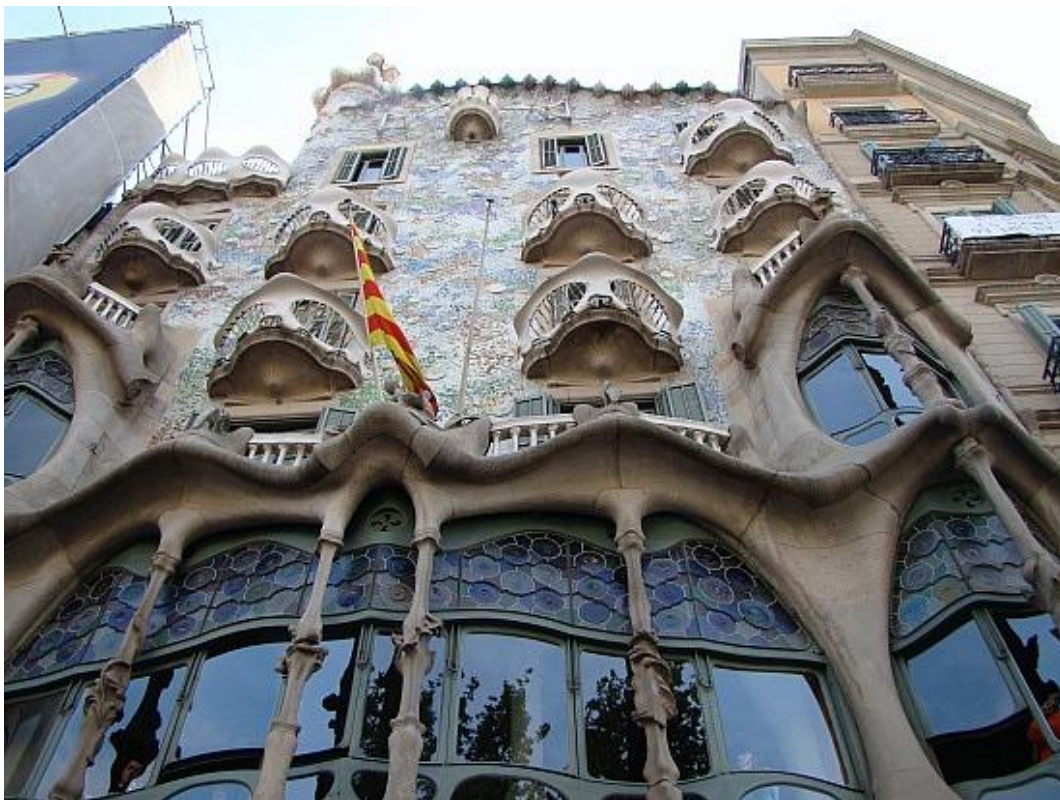
Image 2.11 View from street entrance. (By Author) Accessed 17/11/2008
