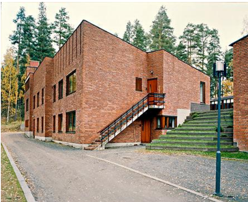
Image 2.7 View into building and courtyard ( URL 009 ) Accessed 15/04/2011
