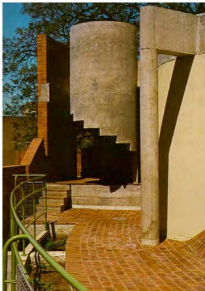
Figure 5.23. View showing well crafted entrance using concrete and brick. (Architect & Builder, 1983).
