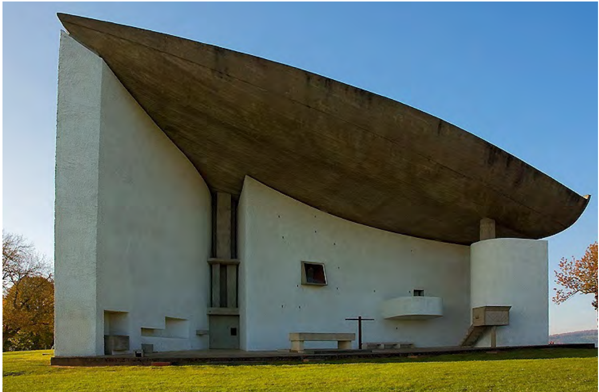
Figure 4.41. View of outdoor sanctuary at Ronchamp (Taillard, 2008) (Web 048).
