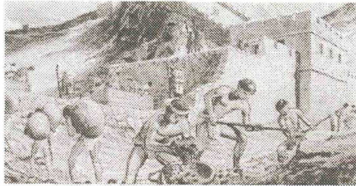
Figure 2.1: A material handler carrying rocks to the building site for the Great Wall of China.[Firth]
