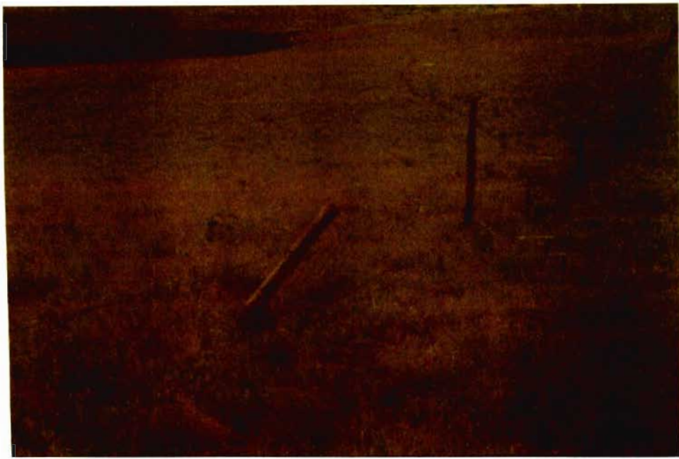
Plate1: Broken fences (fence-line 3) December 2002
