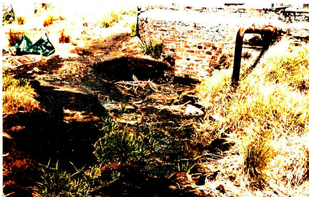
Plate 1a: General view of soil contamination at the project site. The leaking reservoir, containing caustic effluent, is visible in the background.
