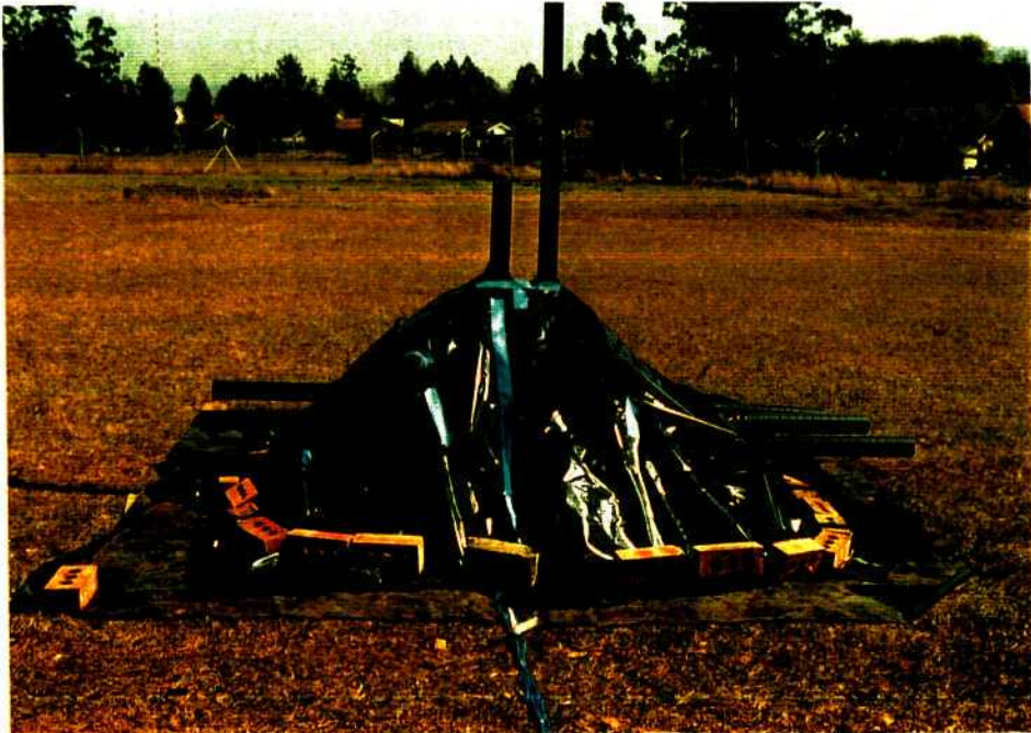
Plate 5b: Side view of the complete biopile. The long vertical riser is connected to the lower pipe array while the short vertical riser is connected to the upper pipe array.
