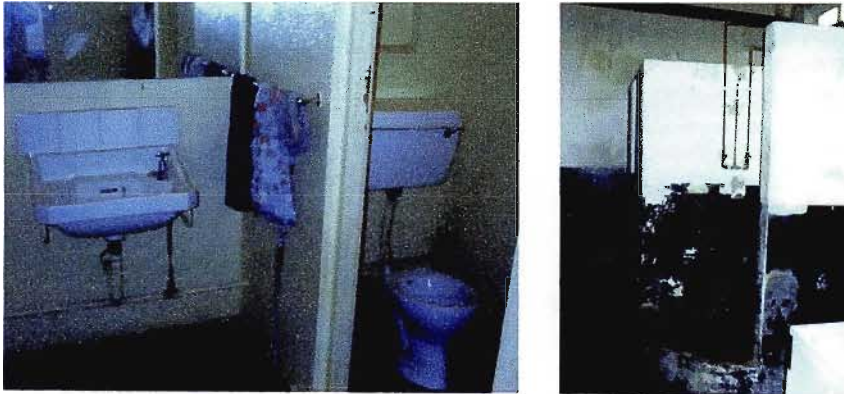
Fig. 11 – Toilet & Shower Facilities in Aliwal Night Shelter
