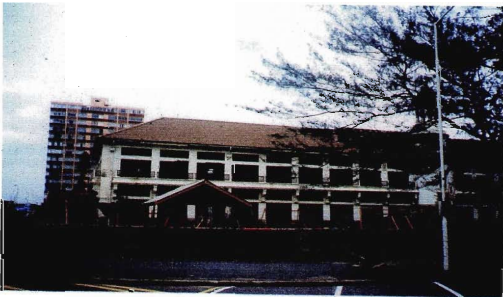
Photograph 7: A building requiring rehabilitation – the Children's Hospital. Location: Taken from South Beach Avenue
