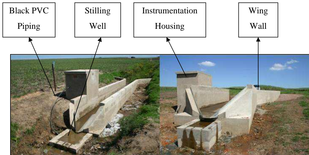
Figure 4.12 Flume 1 (left) and Flume 2 (right) of the Mkabela Catchment
