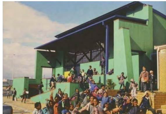
Fig4.13 - Facade responding to street edge (Source: Deckler et al; 2006: 74)
