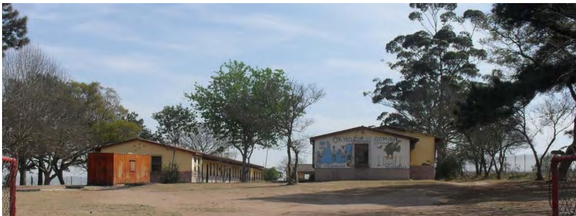
Fig 6.17 – illustrates a typical school in Mpumalanga lacking supplementary services (Source: Author)
