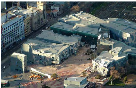
Fig 5.23 – illustrates public space defined by building massing (Source: fedsquare.com)
