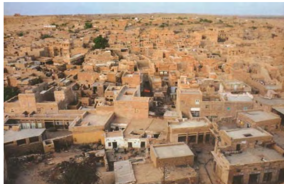
Fig 3.5 – Jaisalmer traditional vernacular dense urban settlement ( Source: Ameen; 1997:54)
