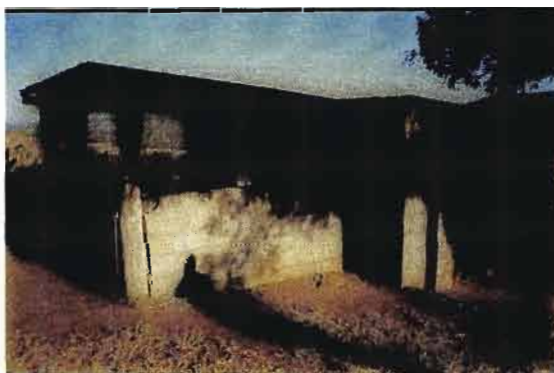
Brick House, Single Milking Parlour
