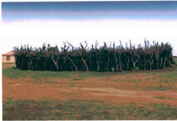
Plate 6.3. A kraal made from laths and poles
