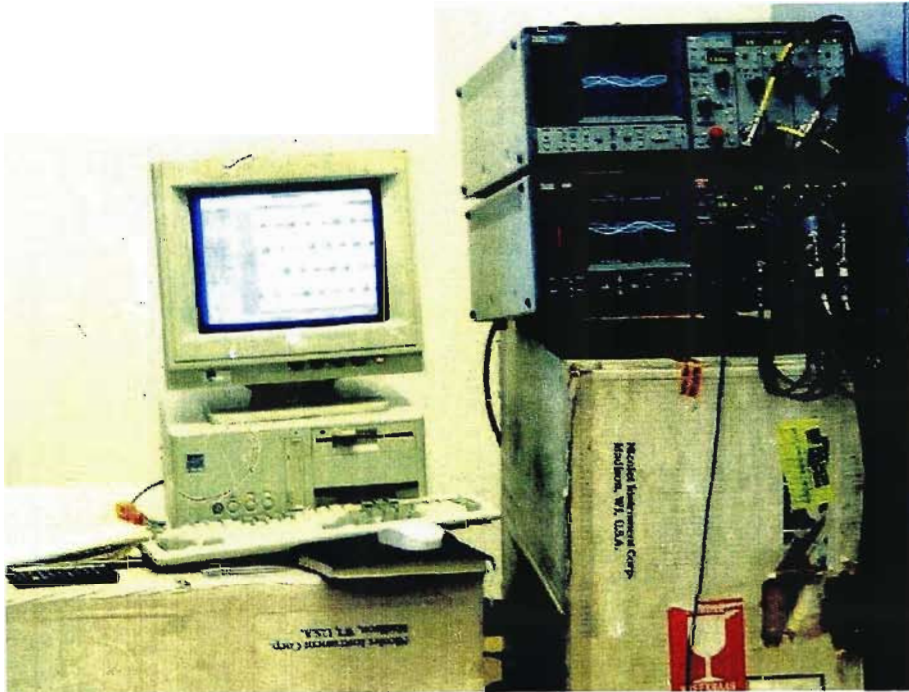
Figure 10.2: Measurement equipment in the Komatipoort substation.
