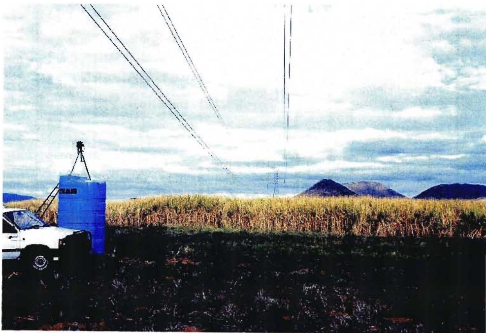
Figure 10. 3: Delta configuration 275kV twin Zebra Transmission Line.
