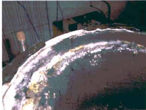
Figure 5-2: Picture of the contaminated insulating layers in the pyrolysis reactor
