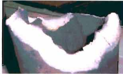
Figure 5-1: Showing the extent of the damaged ceramic used in the feed zone
