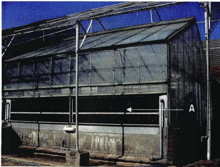
Figure 2.1 Glasshouse used for the rearing of *T. vaporariorum*. A - wet wall cooling system.
